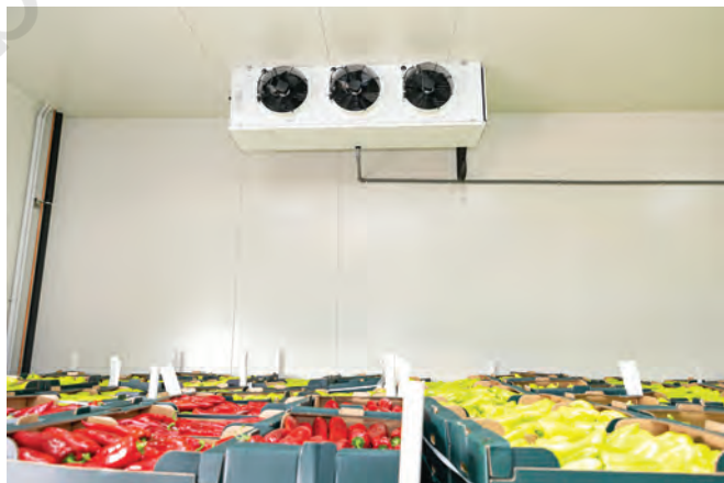
Fig. 12.12. Cold storage facility for vegetables
